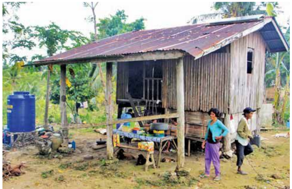
This is the modest home of Obejero where the solar power system and rainwater collection facility was installed.
