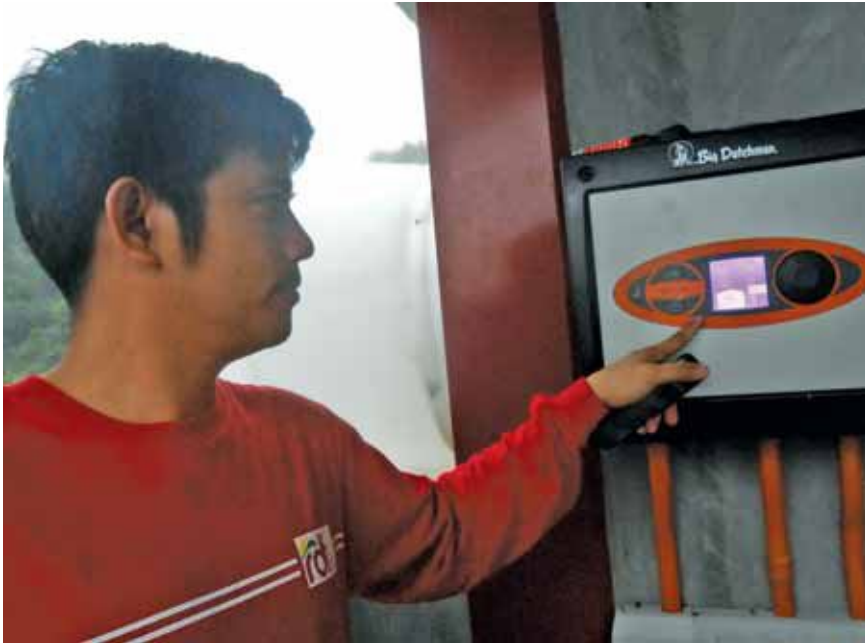
Dr. Peregrino showing the controls of the computer system.
