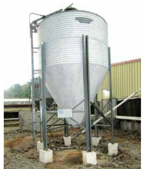
The silo where the feed is stored for automatic feeding.
